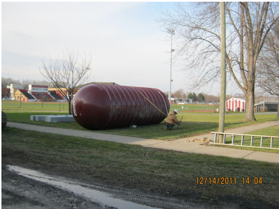
8000 Gallon Fuel Tank for Generator
