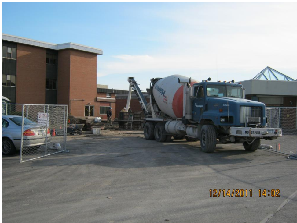
Concrete Placement for Loading Dock Foundation Wall
