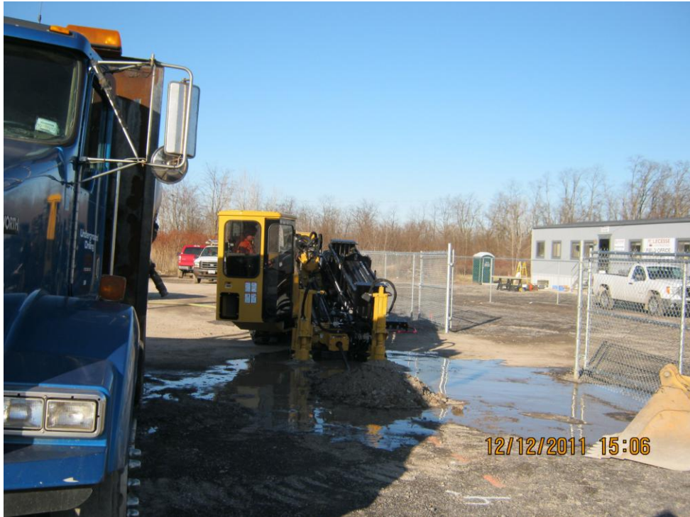
Directional Boring for O-2 Line
