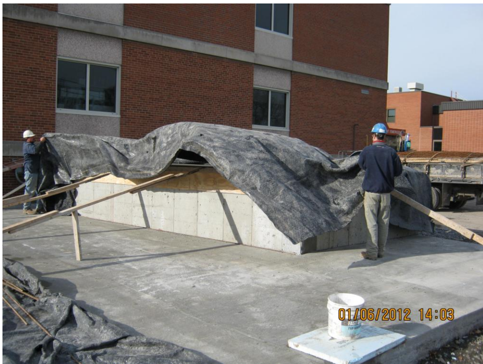
Winter Protection for Trash Dock Floor
