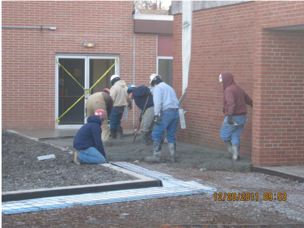
Floor Placement for Temporary Loading Dock
